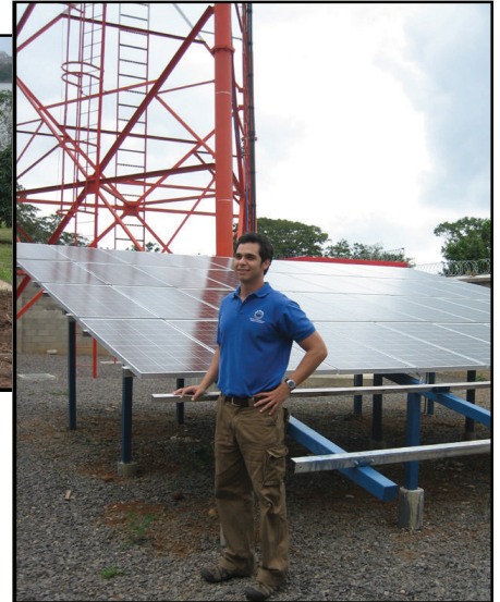
(Above) On Nicaragua's Isla de San Fernando, 30 Kyocera KC130 panels power hotels and homes on the island tourist destination. (Right) ECAMI's Sales Manager Max Lacayo Cortes demonstrates a PV array of 50 KC130TM modules that powers a phone tower in Nicaragua, cutting generator use and thus saving fuel and CO2 emissions.
